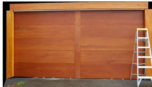
Above: 6 foot wide overhead door ready for trim or siding
